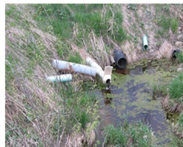
Figure 3 - Plastic tile lines and tile drainage ditch
